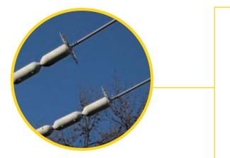
LINE GUARDS (SPINNERS) TransGard recommends the installation and maintenance of line guards on all distribution lines leading out of the fenced in area. Install line guards in a way that will drop falling animals well outside the perimeter of the fence system. Install line guards with line clamps to keep them from sliding toward the fence line. In addition, consider pole wraps that prevent climbing animals from using nearby wooden poles for substation access.
