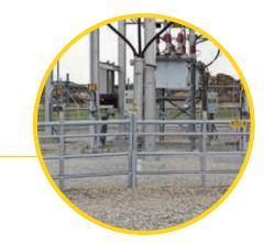
**KEY POINT:** As noted on Page 8, it is important that each panel is installed with one end post resting on a long post and one post resting on a short post of its bordering Galvanized Stands. Another reason for following this step carefully is to ensure the above step to access the substation via any panel.
