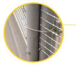
When installing the electrical connections, the lower jumper wire also serves to secure the snake guard in place.
