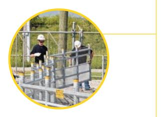
**KEY POINT:** Because the Primary Entryway (and any Secondary Gateways) are in a fixed position, you must start installing the fence at the gateways, and extend in both directions from them. Fence assembly should then proceed by adding panels in each direction from Primary Entryways and Secondary Gateways. The location where the final fence panels will be joined together should offer more flexibility for completion of the fence.
