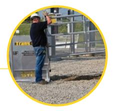
Remove the black cap from the Fence Panel end post at the entryway and install the upper fence bracket into the top of the panel end post.
