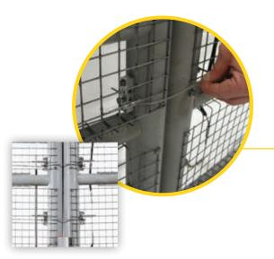
Next, push the jumper wire through the bottom hole of the terminal block on the adjacent panel. INSTALLATION *Electrical Connections*
