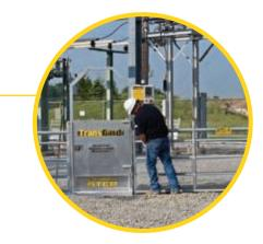
Rake a shallow depression in the gravel large enough to accommodate the base of the Primary Entryway.
