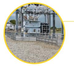
Walk the perimeter of the fence and listen for any snapping noises which would signal a short in the fence from a loose connection or missing Insulator Sleeve.
