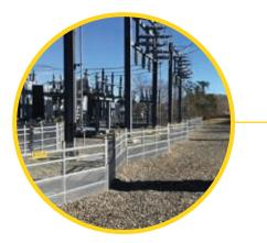
**KEY POINT:** For strength, stability, and easier service access, make sure that each Galvanized Stand faces the same direction around the entire fence perimeter. Then, make sure each panel is resting on both a long and short post of its bordering stands.
